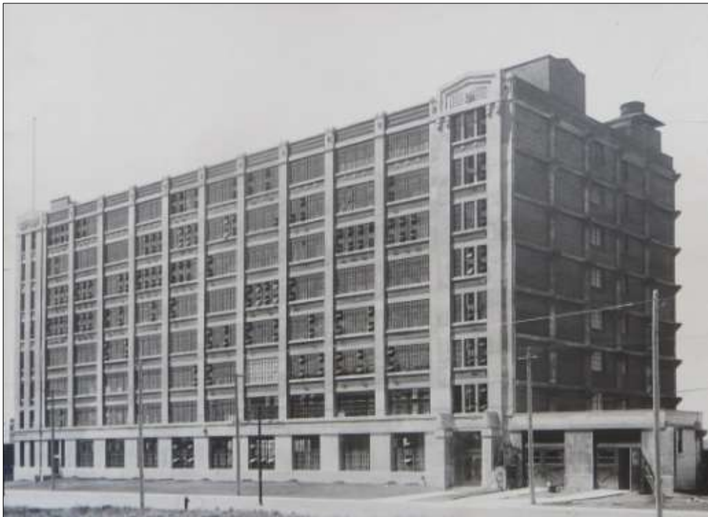
Facing southwest. Probably taken shortly after completion in 1916. Note the projecting concrete supports on the north face for potential future expansion – perhaps adding another section the same size as the existing structure, with the present north entrance then being located in the middle of the larger structure. As well, there is a two-bay single storey structure on the far right that might be part of a garage. This is no longer extant. (Source: Provincial Archives of Saskatchewan: R-B9593)
