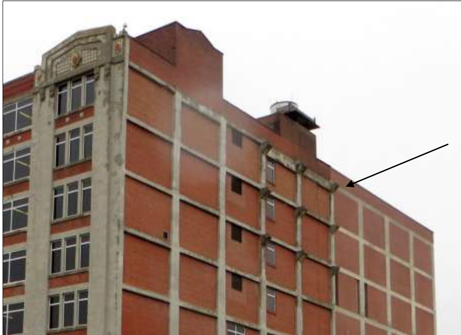
Detail of the additional structural supports built into the upper two storeys of the original 1915-16 north wall.
