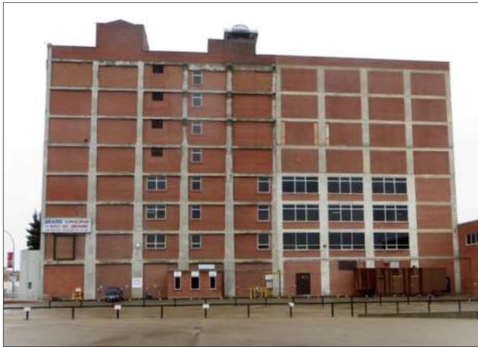
The north wall showing the original 5-bay wide construction on the left and two 4-bay wide additions built on the right. The lower four floors were built sometime between 1922 and 1950; the upper four windowless floors were added after 1950. (Source: Frank Korvemaker, 4 November 2015)
